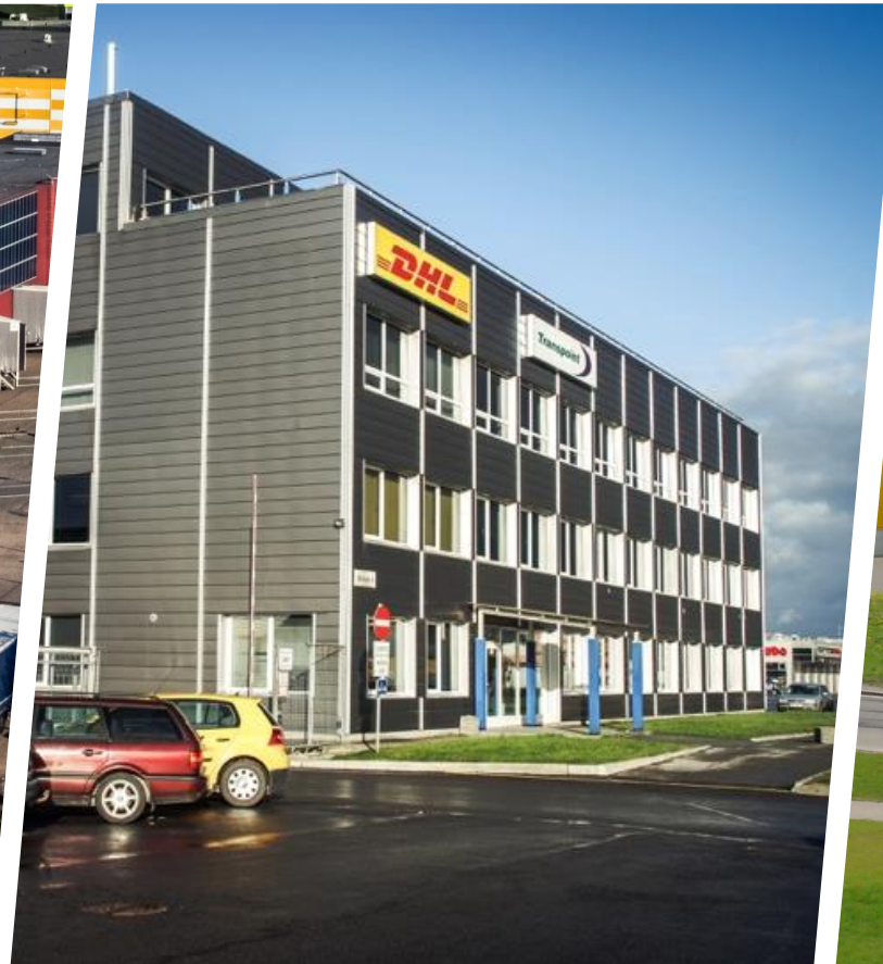
Betooni 6 logistics centre Betooni 6, Tallinn
