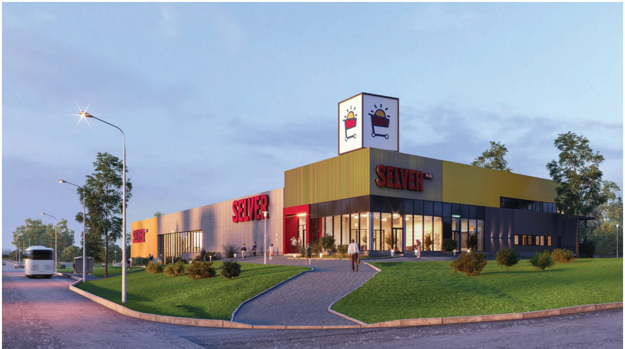
The new Selver store will be completed in December 2017
