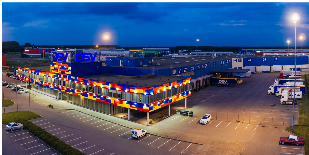
DSV logistics center in Tallinn
